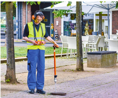
Pre-locating with the SeCorrPhon AC 200
