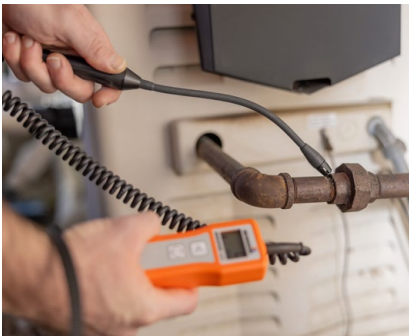
Inspecting a gas pool heating system
