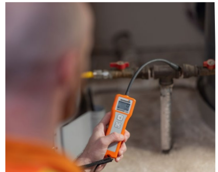
Inspecting a heating system
