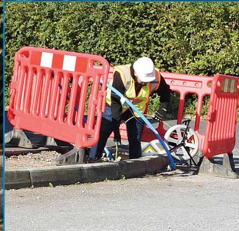
**FlexiTrace** is used with a Schonstedt Pipe & Cable Locator to find and trace small diameter, non-metallic pipes and other non-conductive utilities. The entire length of FlexiTrace can be detected from above ground.
