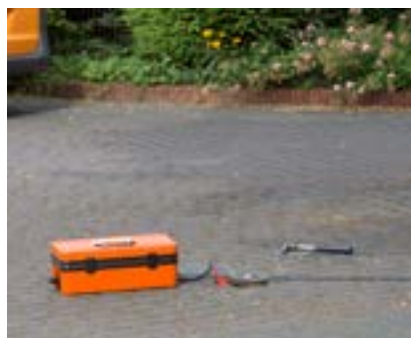
Acoustic location of main pipes
